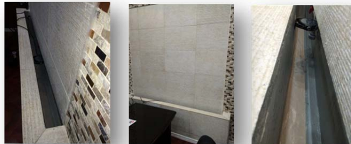
Completed City Hall fountain trough restoration
