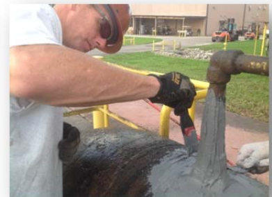
Applying the first coat of MCOR 3115
