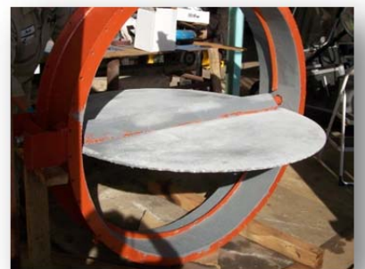
Steel surface restored in its entirety
