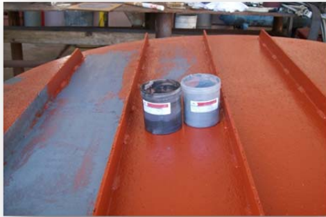
Filling in pits and resurfacing metal with MCOR ™ 3115 | mClad ™ mFill ™
